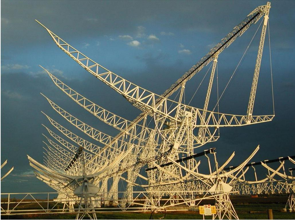
**Figure 2.3: The E/W antenna is the largest arm of the Cross telescope**
