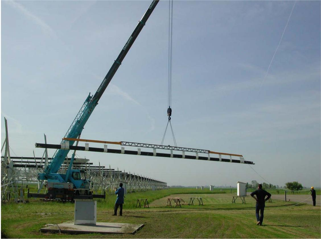
Fig. 2.2.2 Uninstalling the focal line from a cylindrical reflector
